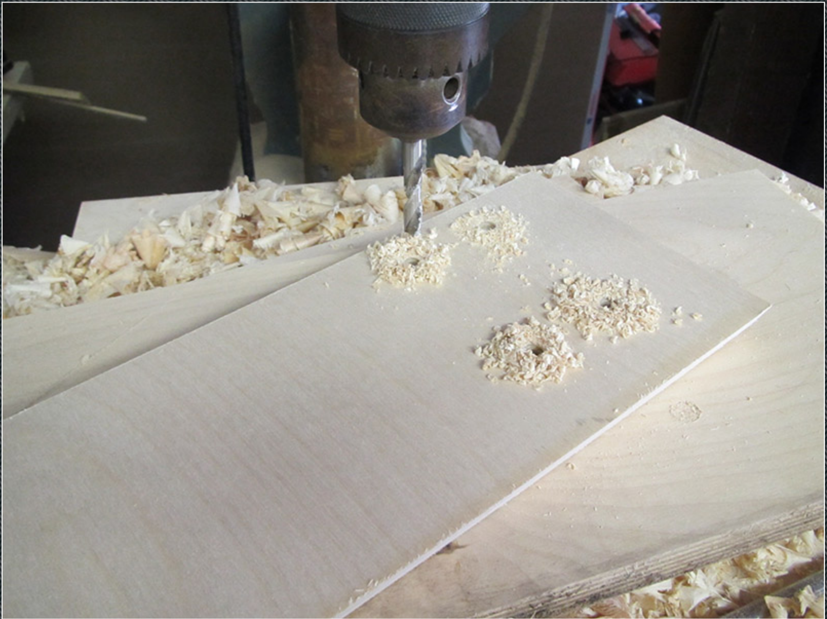
Drilling the holes for the 1/4-20 hurricane nuts that the casters will bolt to. The same type nuts are used for the towel bar.
